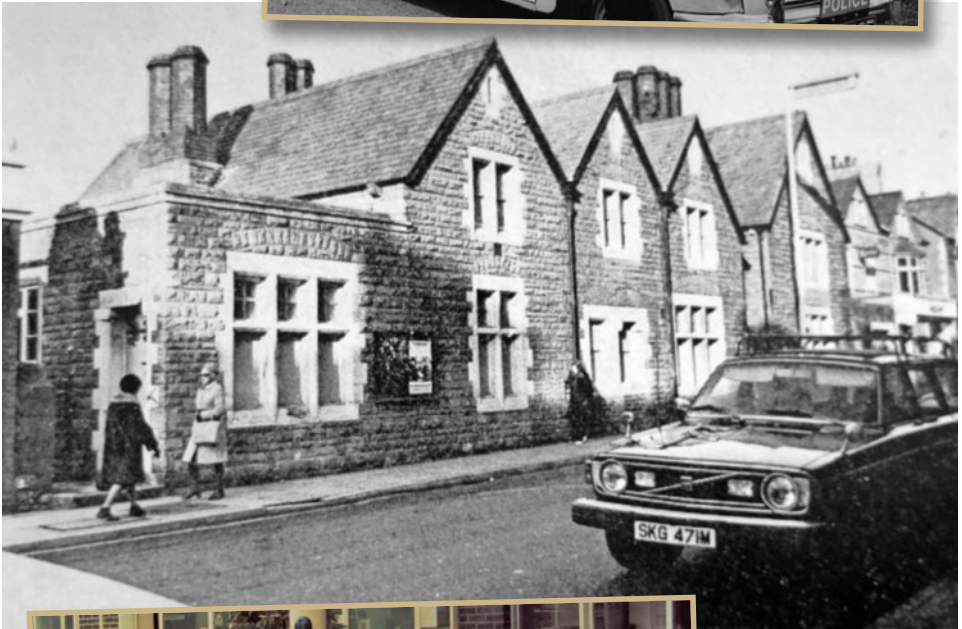
The old Porthcawl Police Station, built in 1881.
